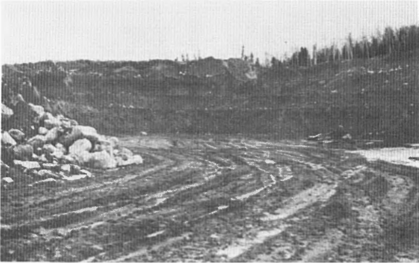
A — Excavation in boulder clay along access road to Cassé lake.
