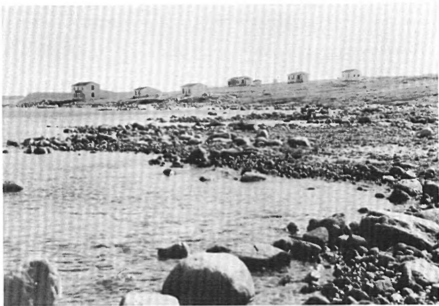
B - Port Harrison post on Hudson Bay. (Photo, Hudson's Bay Co.)
