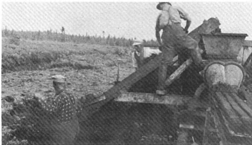
Plate XVI—"Quebec Type" peat fuel machine in operation at St-Lambert, Lévis county.
