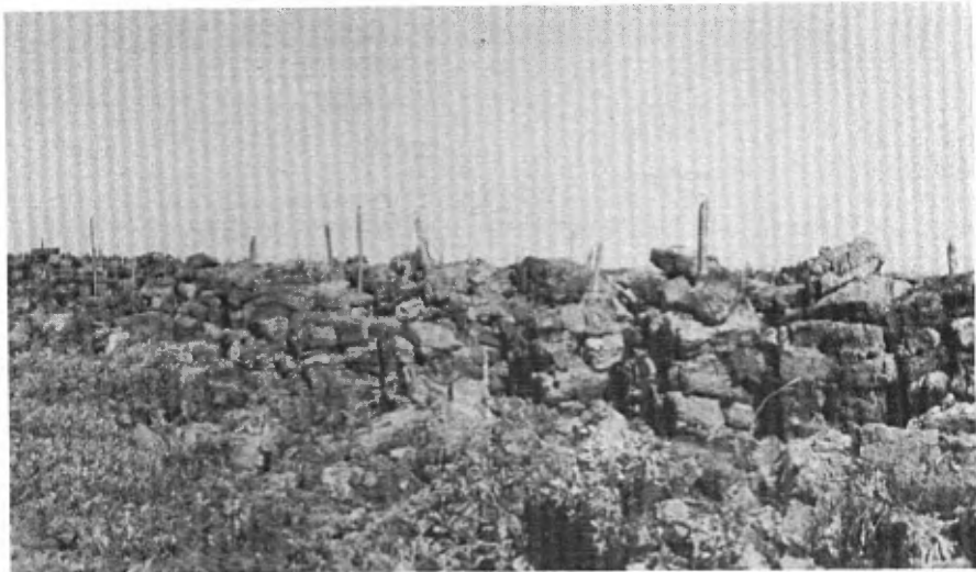
Plate XI—Method of drying peat blocks at the St-Anaclet bog, operated by Henri Reid.
