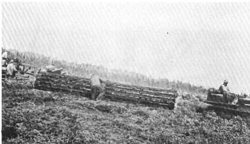
Plate XVII—Caterpillar tractor used in spreading and harvesting peat fuel.
