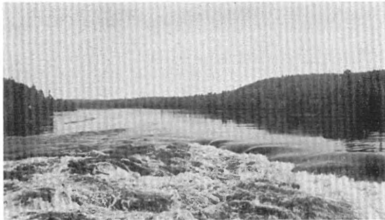
B.—Gatineau river, looking upstream from the bridge on the Mont Laurier-Senneterre highway (boundary of Sicotte and Lytton townships).
