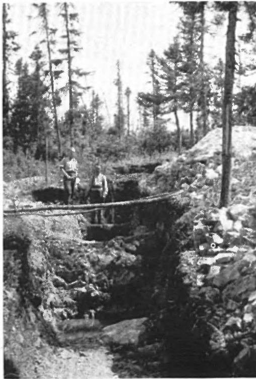
B.—Trench opened in a serpentine outcrop in search for chromite. Lot 11, range IV, Awantjish township.
