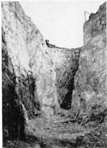
A.— Pit B Canadian Refractories Limited, showing narrowing of ore zone to north.
