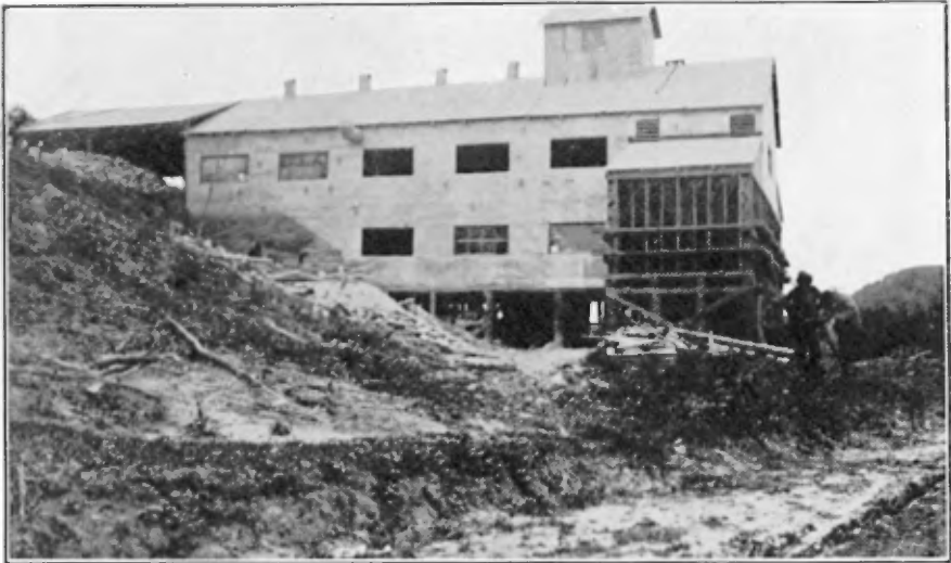
B.—Recently-erected mill, McLean and McNicoll Ltd. property.
