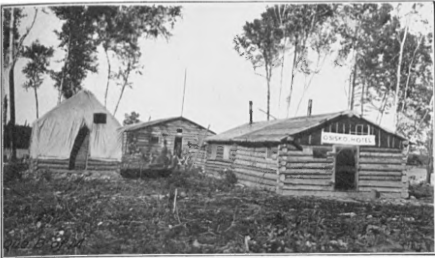
Osisko Hotel, and general store in background, Rouyn townsite, September 1924.
