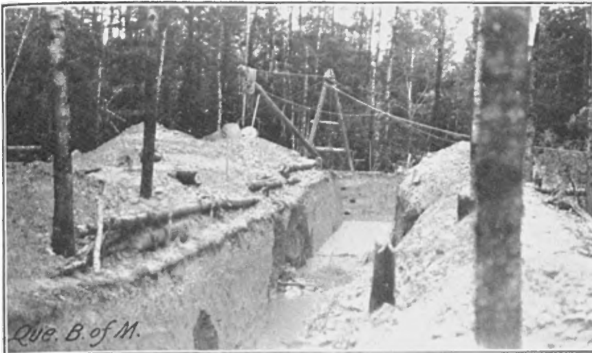
Rouyn township, Sheldon claim.—Trenching in heavy overburden of stratified clay.
