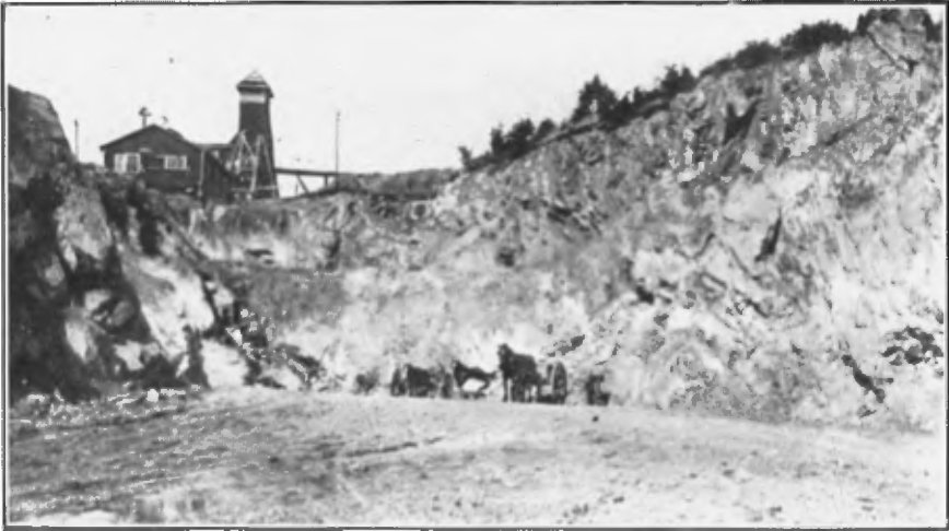
J. V. BELANGER MINING Co., LTD.— Chrome deposit in Coleraine township, worked by quarry method.
