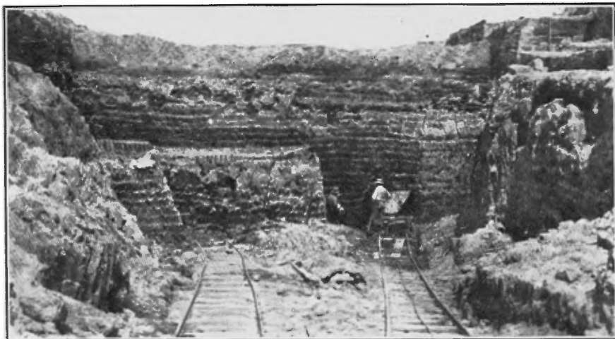
LA COMPAGNIE DE TUYAUX DE DRAINAGE, LTEE.— Clay pit at L'Islet Station showing method of working
