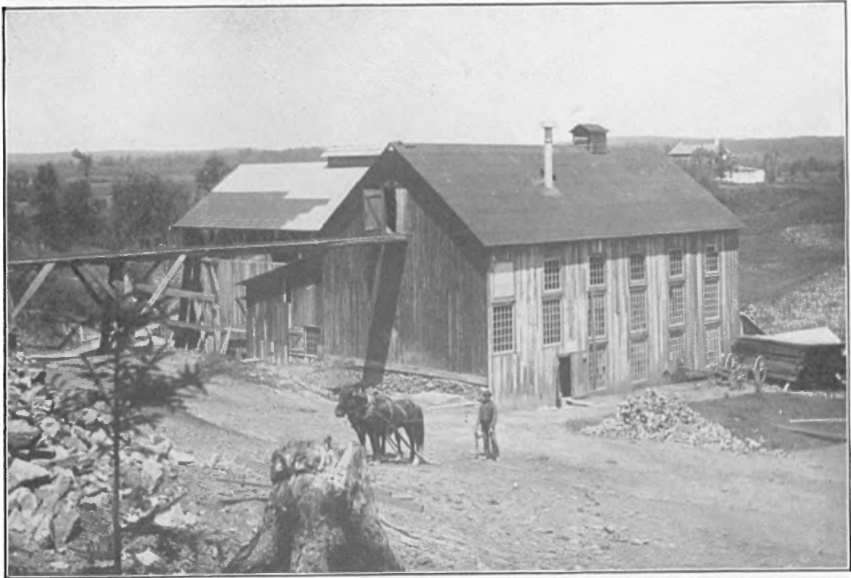
GRAPHITE. —BELL GRAPHITE Co. —Concentrating plant.
