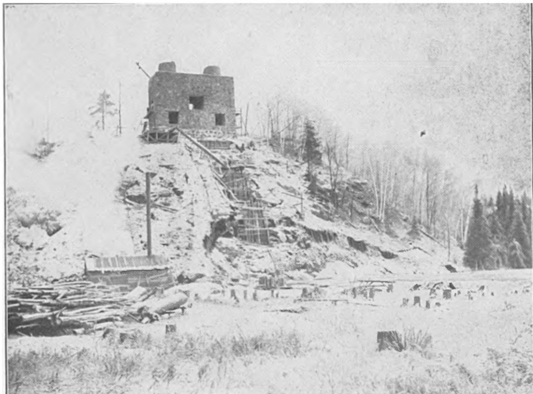
GRAPHITE.—DOMINION GRAPHITE Co.—Drying kilns in course of construction.
