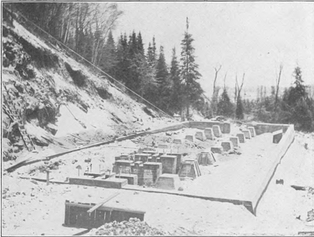
GRAPHITE.—DOMINION GRAPHITE Co.—Foundation of new mill at Stewart Mine.
