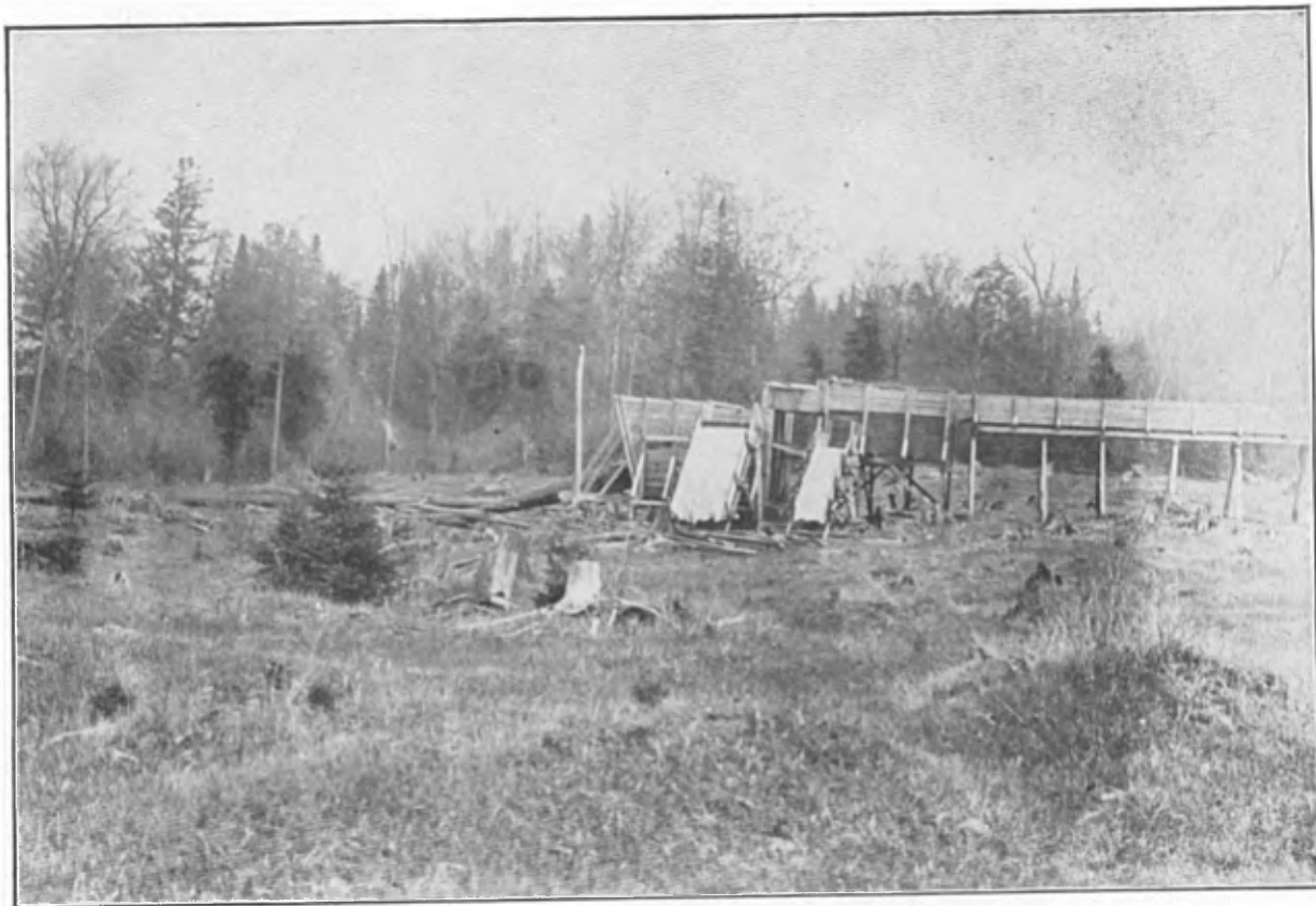
GOLD. —DOMINION GOLD FIELDS, LTD. —Penstock and 18 inch pipe line.
