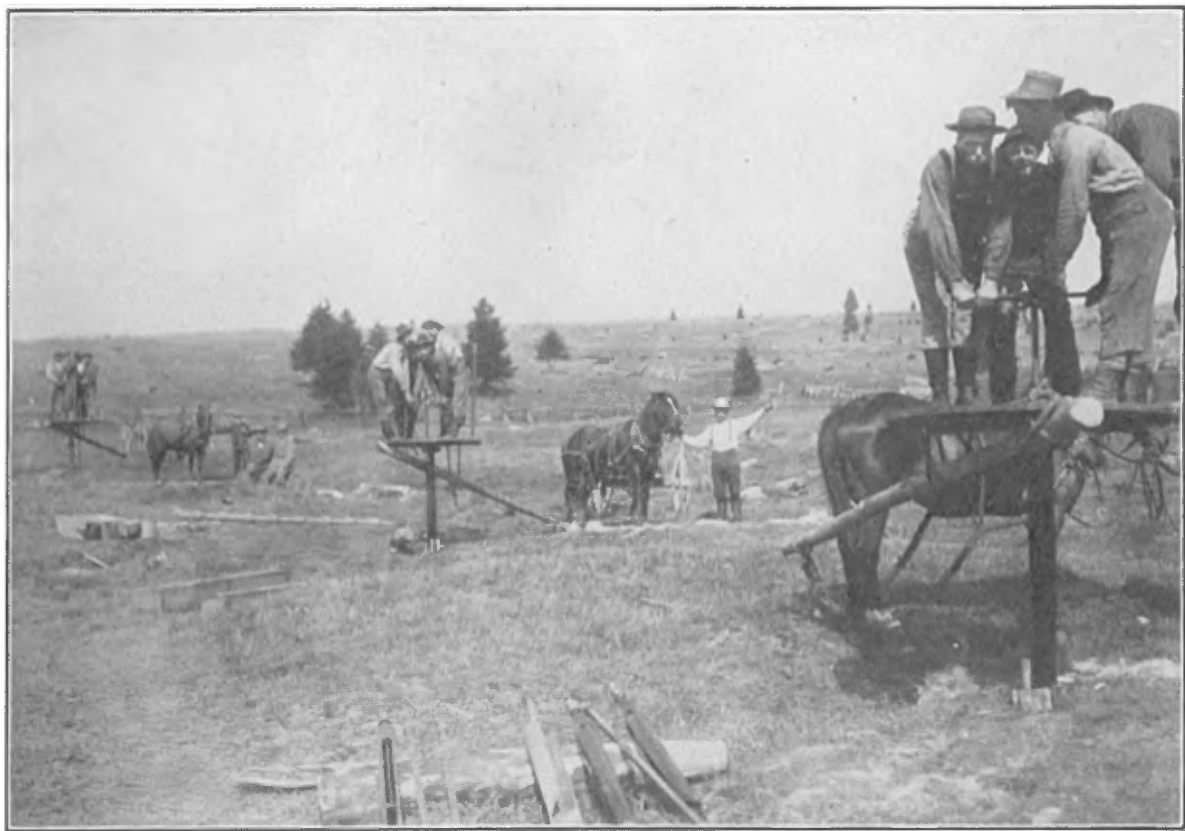
GOLD.—Testing alluvial ground on Gilbert River with Empire drills.
