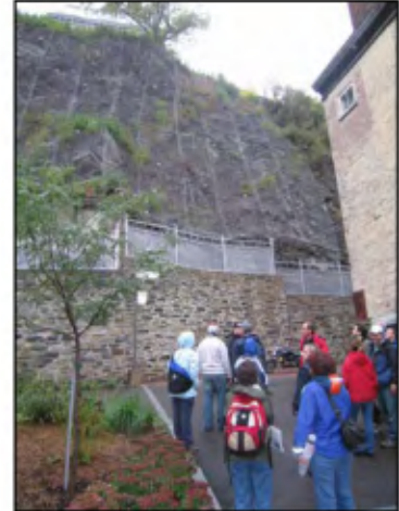
Figure 35. The lane between rue Sous-le-Cap and rue Sault-au-Matelot is now blocked and fencing was recently installed to prevent accidents connected with the landslide hazard. Draped wire mesh, rock bolts and fences installed in the cliff along rue Sault-au-Matelot serves as a reminder that the Place-Royale sector of Cap Diamant is unstable. Corrective work was carried out to make the site safer, including the removal of unstable boulders, the construction of a retaining wall (rue Sault-au-Matelot) and the installation of rock bolts.
