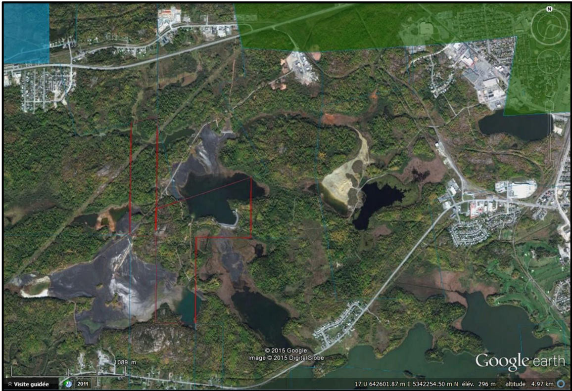
Photo 1. Noranda 5 infrastructures; property outlined in red.
