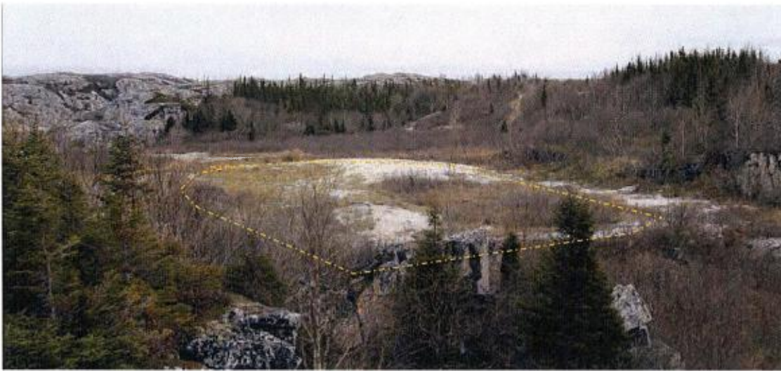
Spar Mica storage facility foundations and residual concentrate. Looking north
