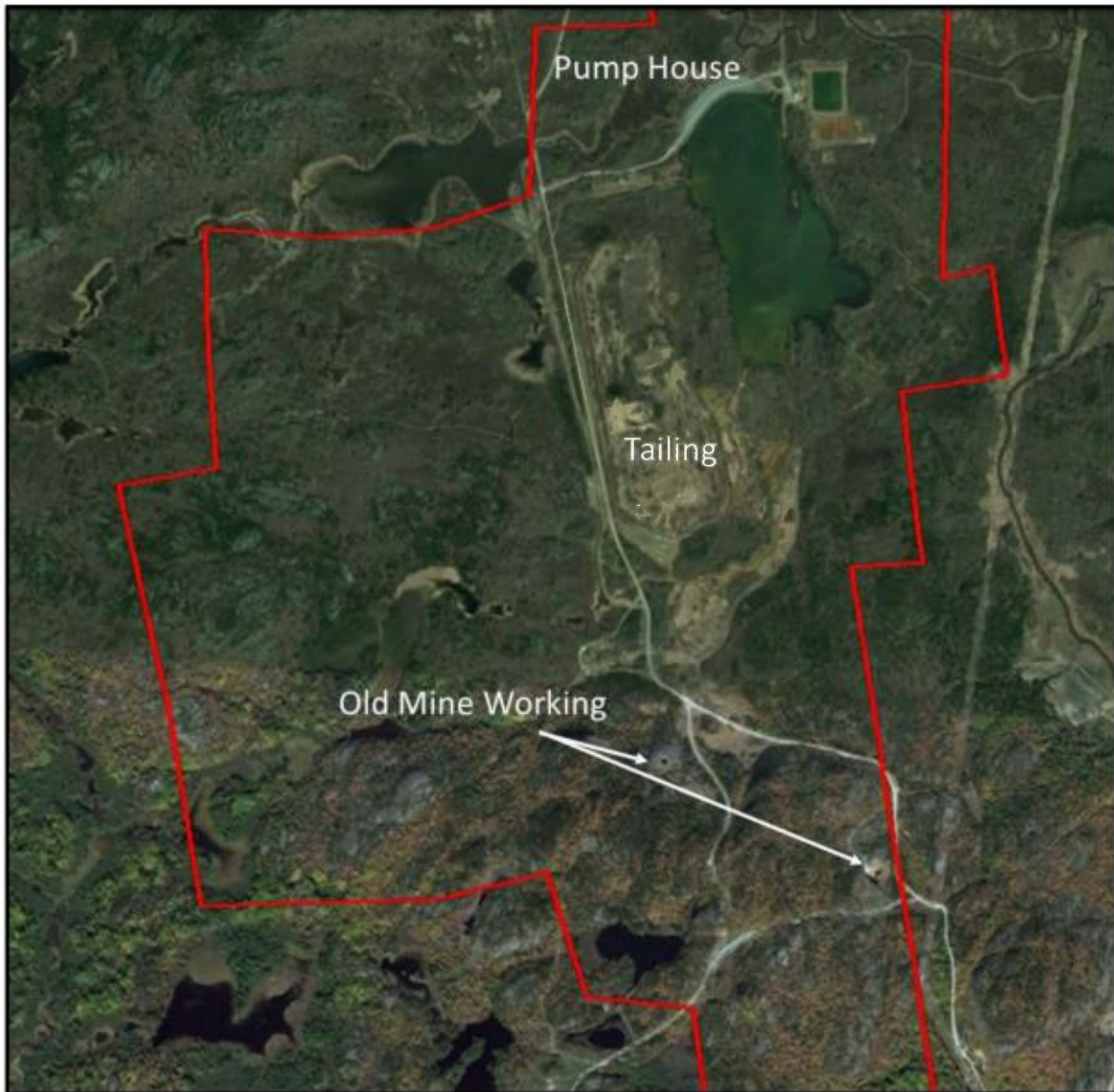
Photo 1. Waite-Amulet remaining infrastructures.
