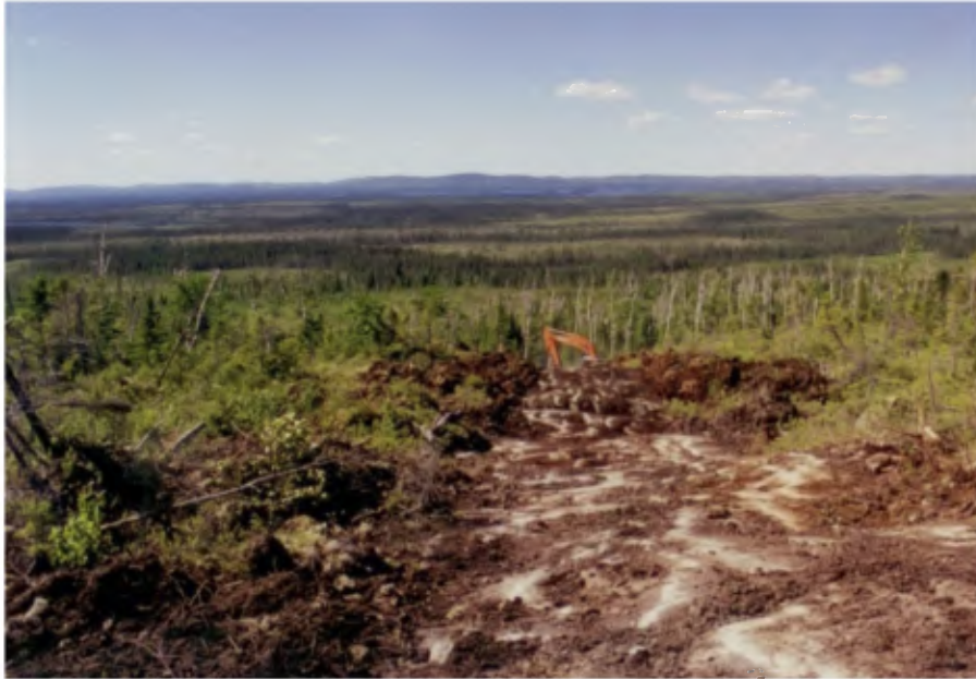
Picture 6: Mechanized stripping done for McKenzie Bay in 1997.
