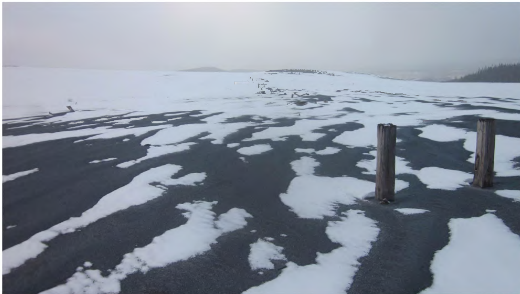
Plate 7: Remnant pipeline trestle support structures across Lac Jeannine Lake tailings pile
