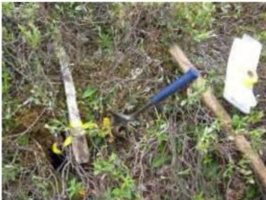
Wood stick identification and rod steel anchor
