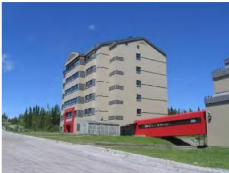
Photo 5.1 – Hydro-Québec Complex Installation at Radisson
