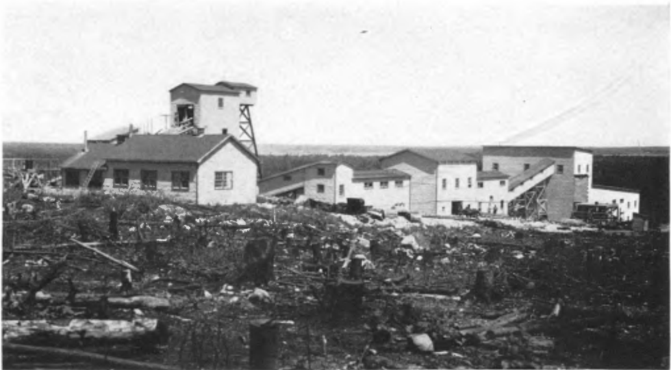
B.—Mill of Molybdenum, Limited, Preissac township. Headframe for 20-degree adit at left, July 1943.
