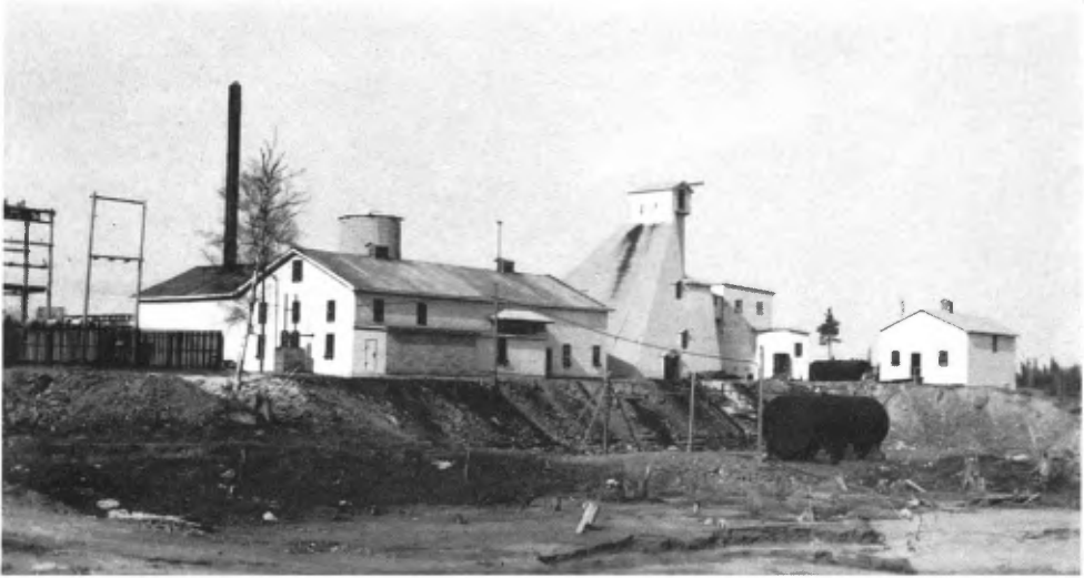
A.—Belleterre Quebec Mines, Limited No. 2 shaft, April 1942.
