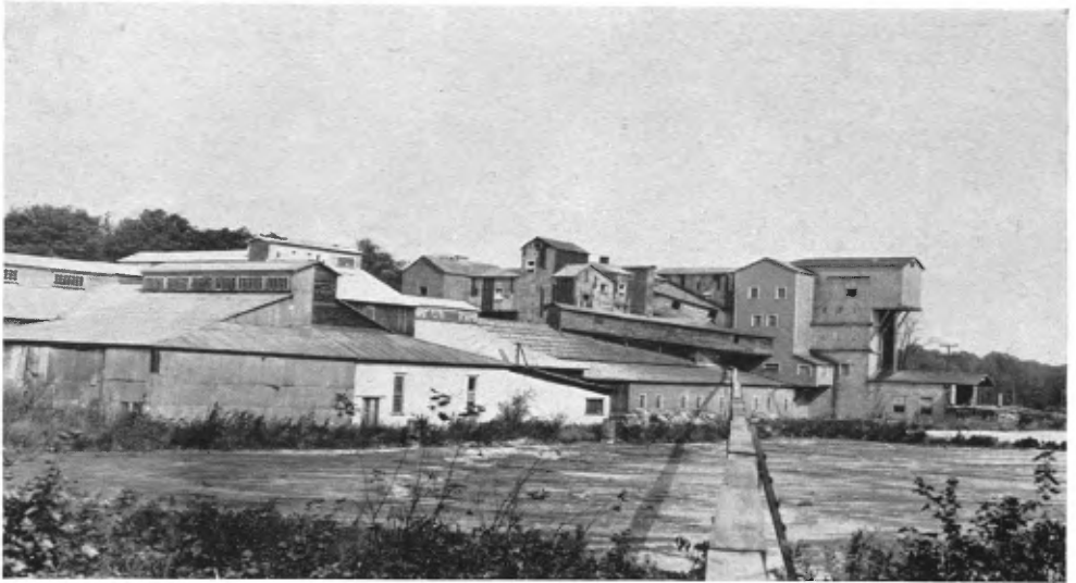
B.—The mill of the Canadian Carborundum Company, St-Canut, Deux-Montagnes.
