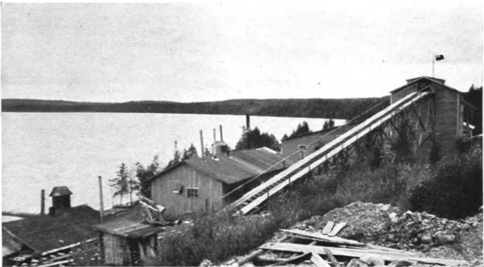
B.—Power House and 25-ton mill of the Lake Rose Mines, Currie Township, August 1938.
