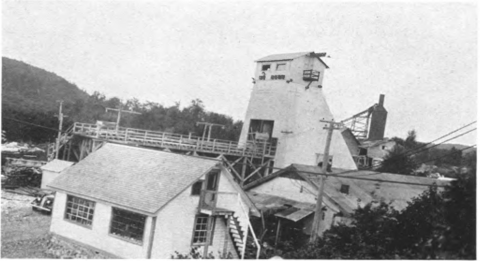
A.—Canadian Refractories Limited, Kilmar, Argenteuil County. Headframe of the shaft.
