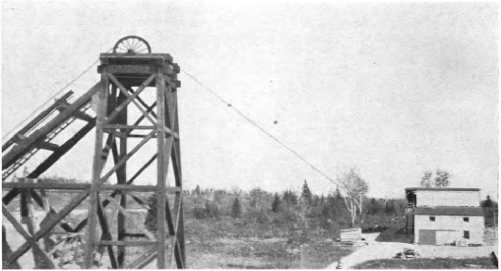
A.—Mill of the Francoeur Gold Mines in Beauchastel Township, August 1938.
