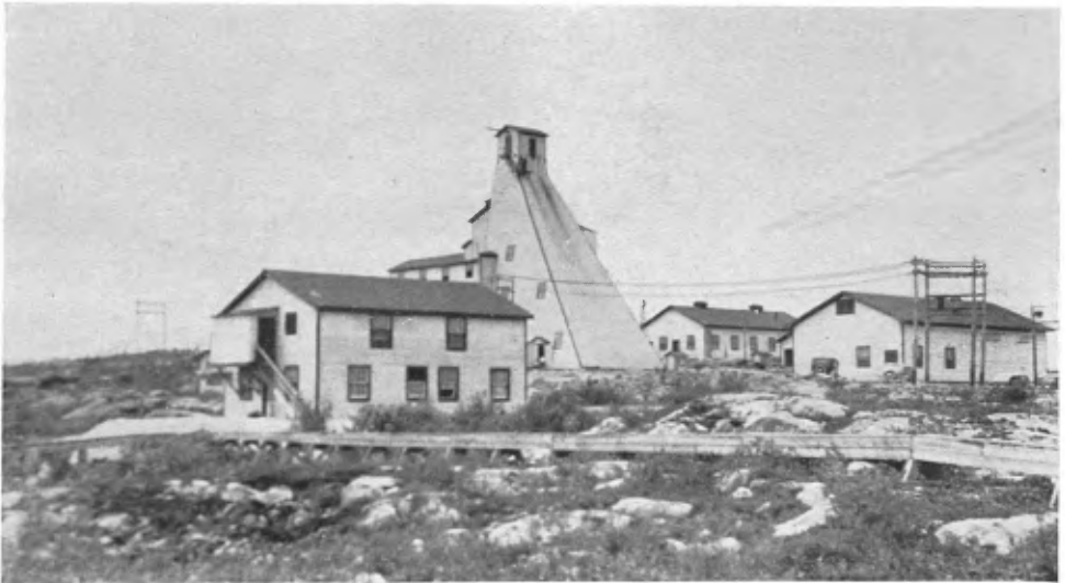
B.—Powell-Rouyn Gold Mines, Rouyn Township. Headframe of the shaft, July 1938.
