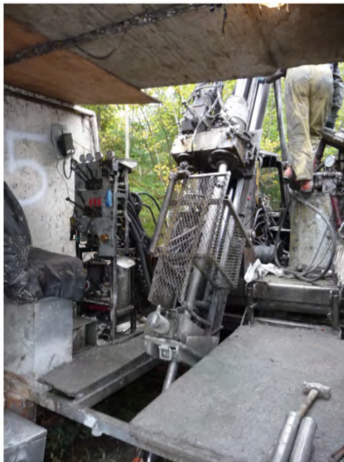
Hole AL-10-08 drill setup
