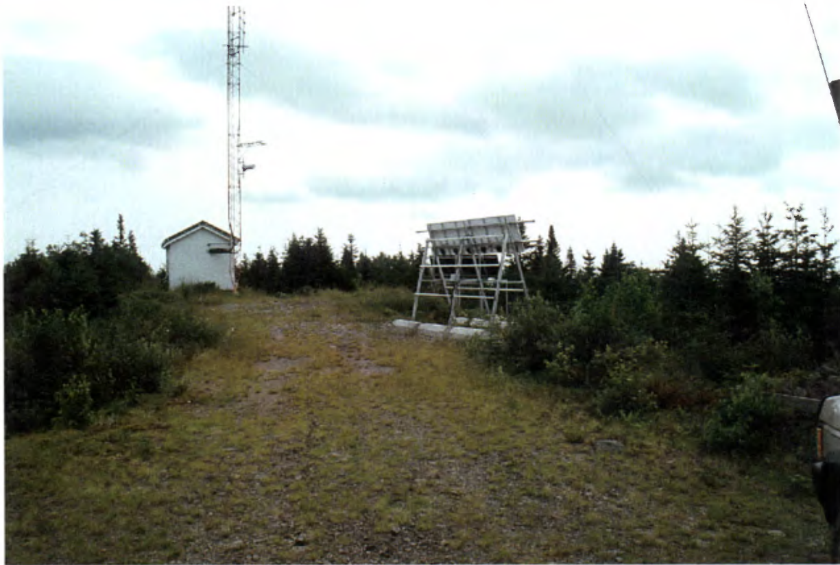
Facilities at the top of Mont de l'Observation
