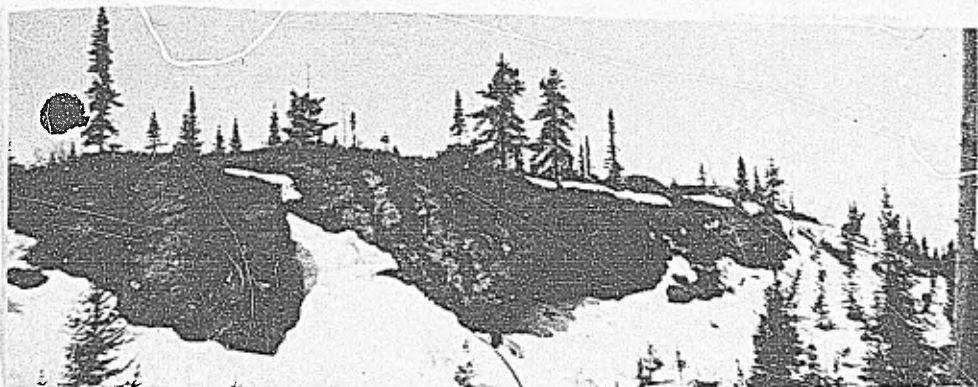
20 - 23 Trenching and stripping bedrock (mica-gneiss), near the north boundary of the property (top). Gneiss outcrops (center and bottom). Cutting the baseline through a heavy growth of spruce.
