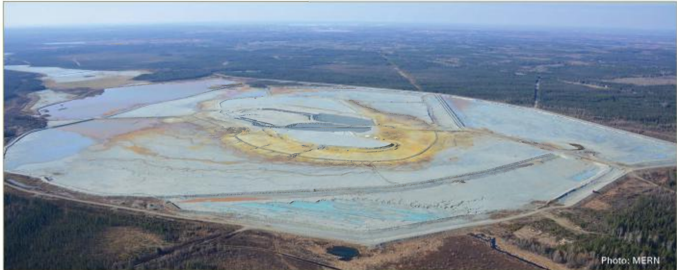
Tailings pond at the Manitou site undergoing rehabilitation work.
