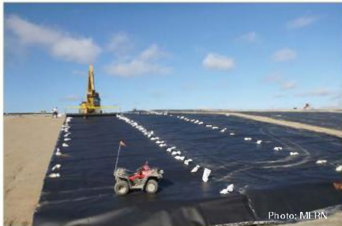
Installation of the geomembrane at the Barvue site.
