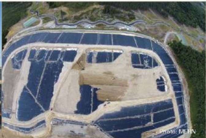
Rehabilitation work at the Barvue site.
