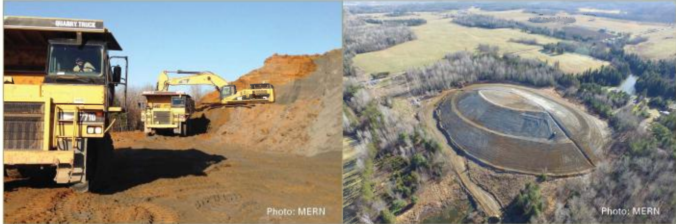
Excavation of mine tailings at pond B.
