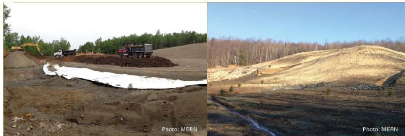
Beginning deposition of waste rock in the containment cell.
