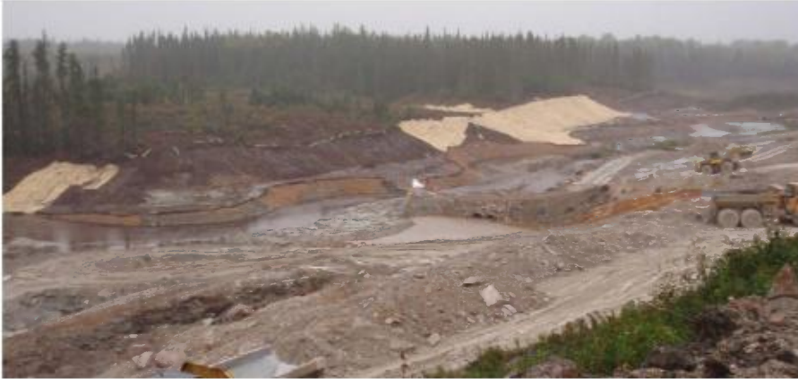
The Barvue site, creek diversion work.
