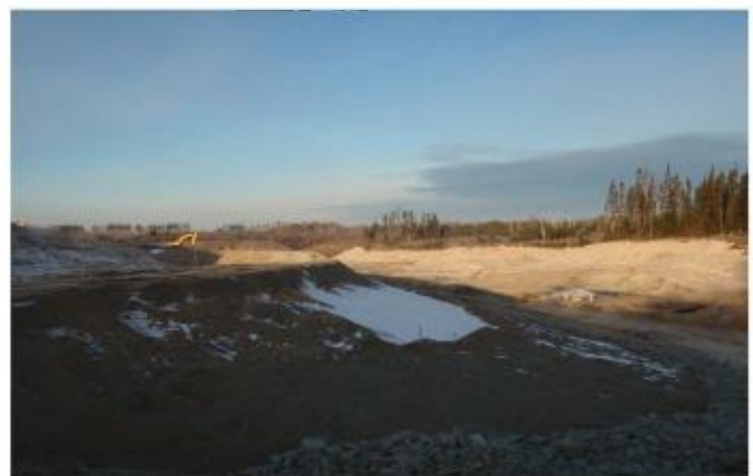
The Barvue site, berm construction.
