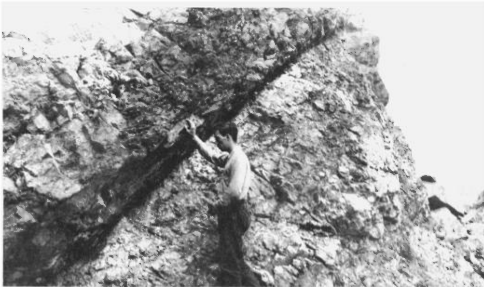
Fig.5 : Fault near the power-house at LaTuque. Looking south.
