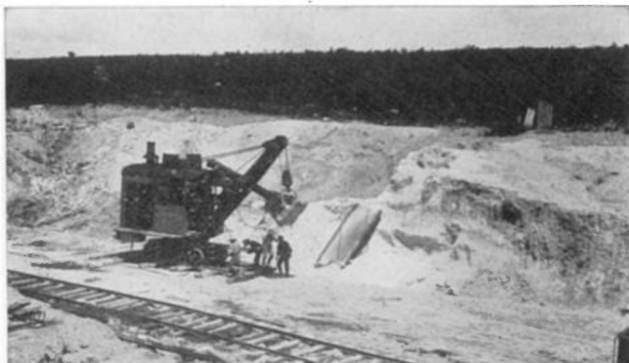
Removing overburden from a deposit of china-clay in Amherst township.
