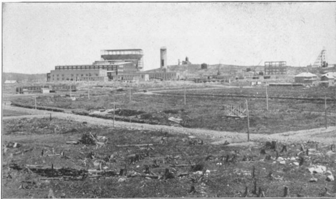
Horne Copper Corporation Ltd.—Noranda smelter in construction at Noranda. Head frame of Horne mine at extreme right
