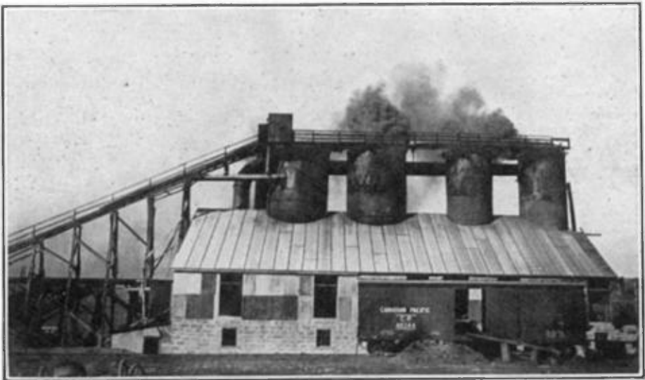
A battery of modern lime kilns at Deschambault.
