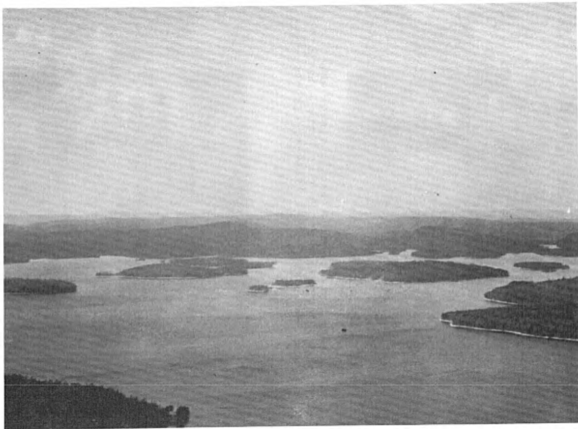
Westward view of the Gouin reservoir from Tower 67.
