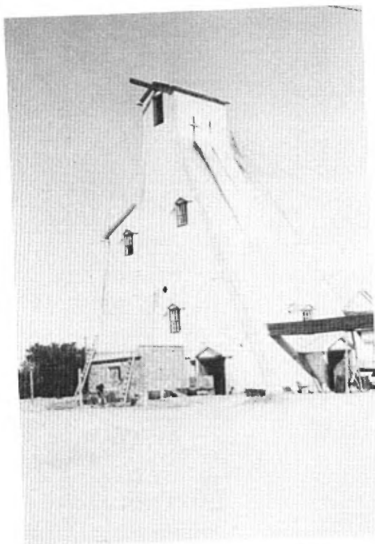
(A) No. 3 shaft, Belleterre Quebec mine.
