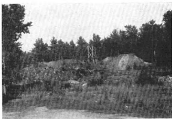
A.—MacDonald shaft, Calumet Mines, Limited. Principal underground work is in this vicinity.
