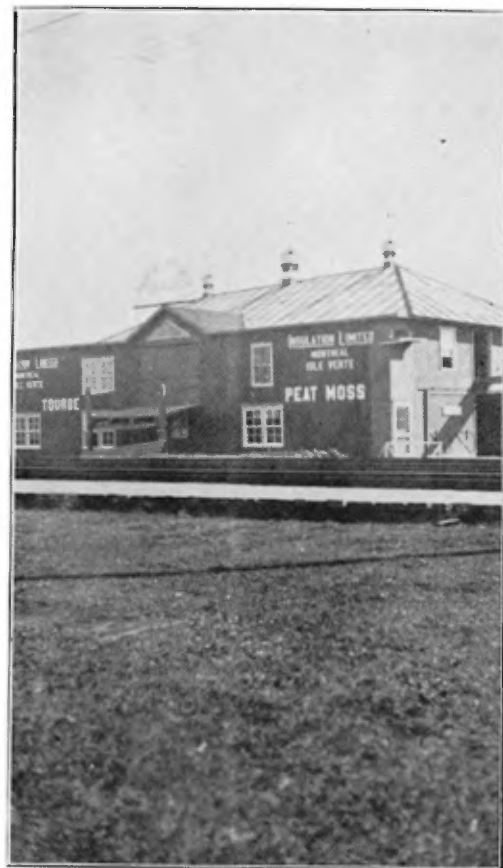
B.—The place of Insulation Limited at Isle Verte, P. Q.
