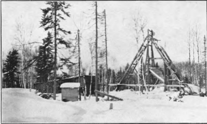
A.—Normont mine shaft, Beauchastel township.
