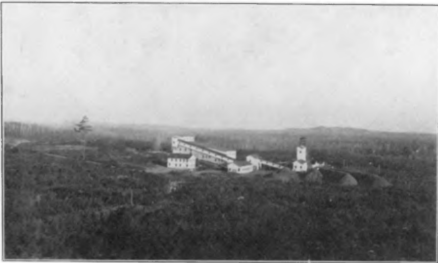
Aldermac mine and mill.
