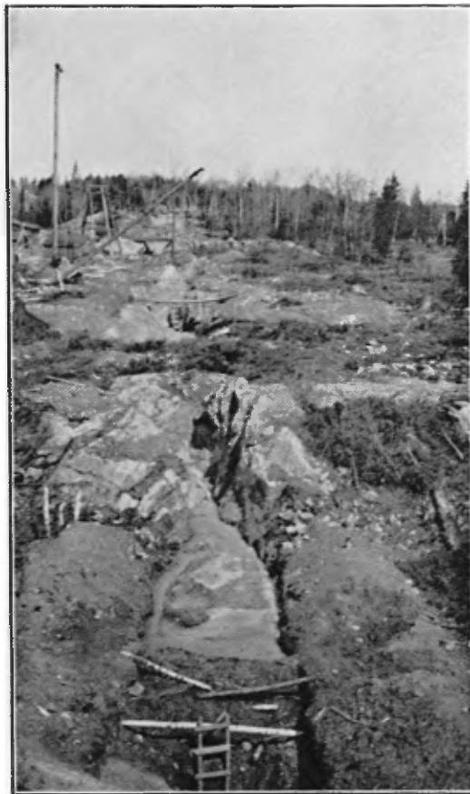
B.—Surface work along the strike of chromite deposit at Sterrett mine, lots 7 and 8, range X, Cleveland township.
