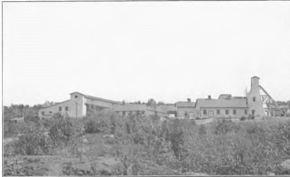
View of the shaft and mill at Granada mine
