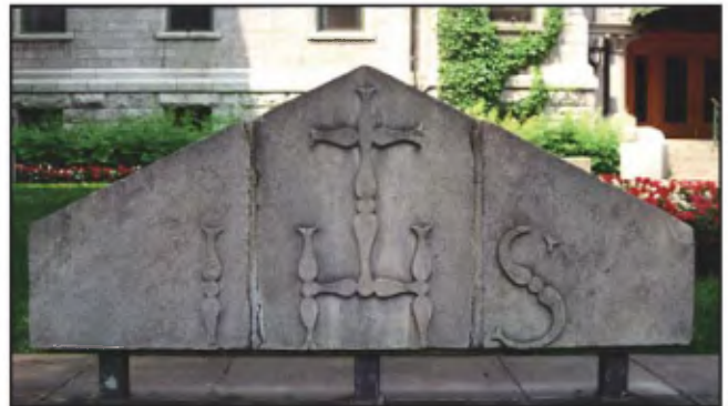
Memorial stones of the Old Jesuit Collège in limestone of the Deschambault Formation from Pointe-aux-Trembles.
