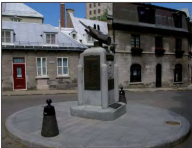
Monument dedicated to teaching nuns with pedestal in Stanstead granite and cartouches in Prairie Green granite.
