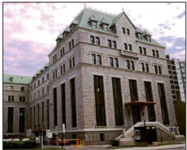
Guy Fregault Building: walls in Saint-Sébastien grey granite; window frames in Deschambault limestone from Saint-Marc-des-Carrières; basement in grey-pink granite from Rivière-à-Pierre..
