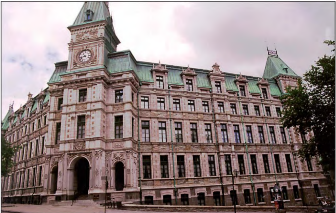
Quebec Old Court House in grey and green sandstones of Cap-à-l'Aigle Formation from La Malbaie, limestone of Deschambault Formation from Saint-Marc-des-Carières, Sillery sandstone of the Chaudière nappe, and Stanstead granite.
