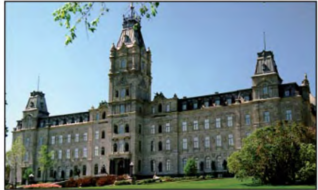
Hôtel du Parlement main facade in Deschambault limestone from Saint-Marc-des-Carrières. Basement is in "Caledonia" granite from Rivière-à-Pierre.
