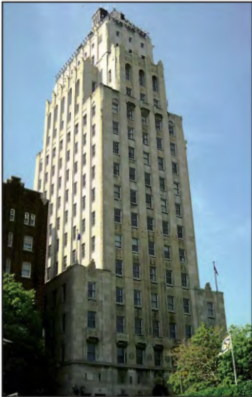
Price Building, faced in part with Deschambault limestone from Saint-Marc-des-Carières, in part with Queenston limestone from Ontario.
