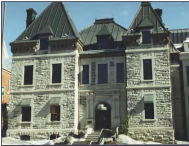
333, Grande Allée Est: Building in Beauport or Château-Richer limestone blocks, and trim in Saint-Marc-des-Carrières limestone.
