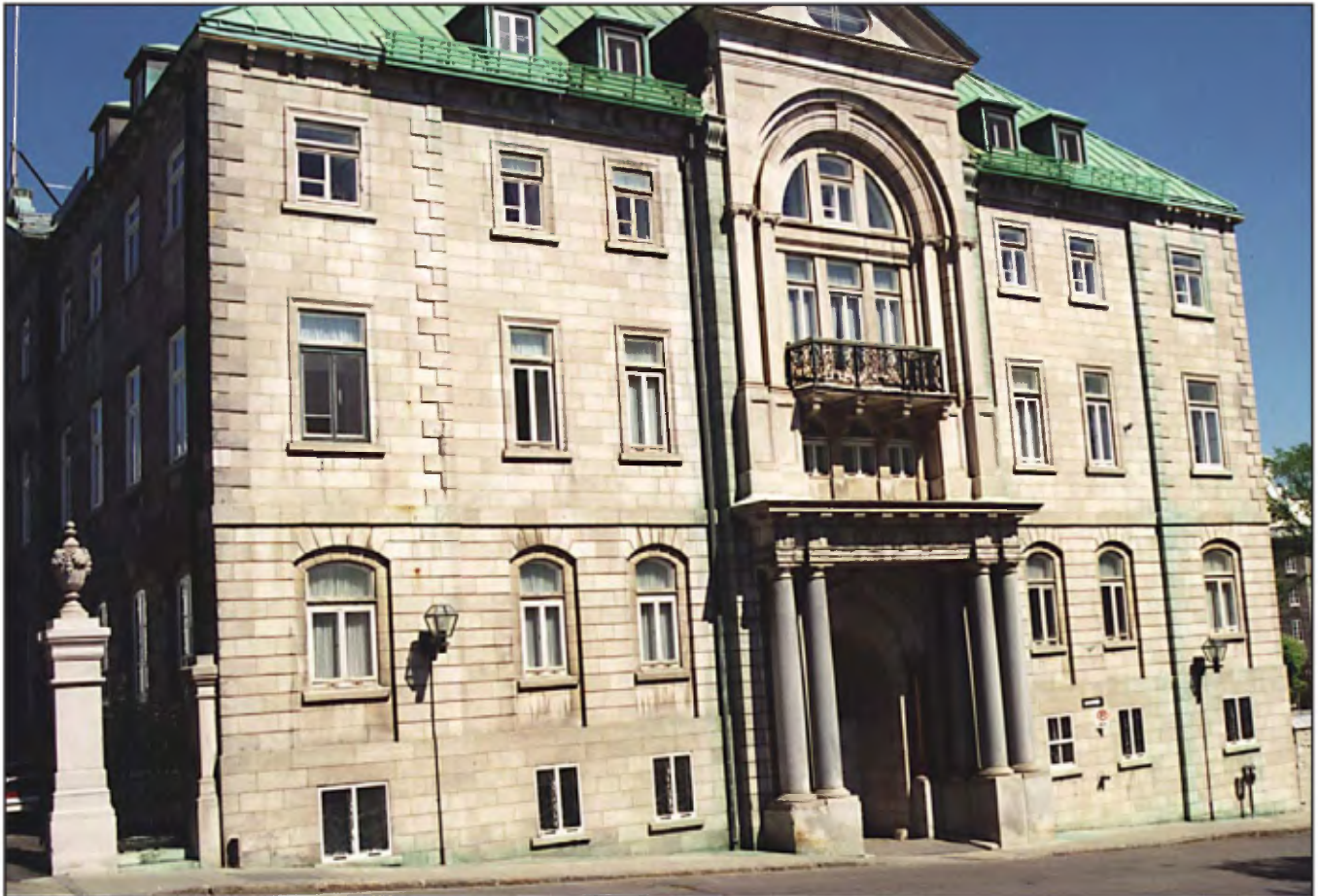
Quebec Archbishop Palace in limestone of Deschambault Formation from Pointe-aux-Trembles and Saint-Marc-des-Carières; columns in grey granite from Stanstead and red granite from St. George, New Brunswick.
