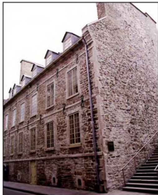
Facade of Maison Estèbe in Ange-Gardien sandstone and trimming in Pointe-aux-Trembles limestone.
