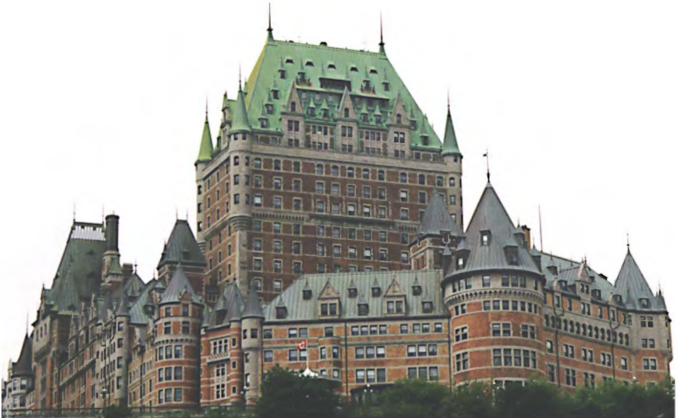
Château Frontenac built in part in Deschambault limestone from Saint-Marc-des-Carières and also in Chazy limestone.
