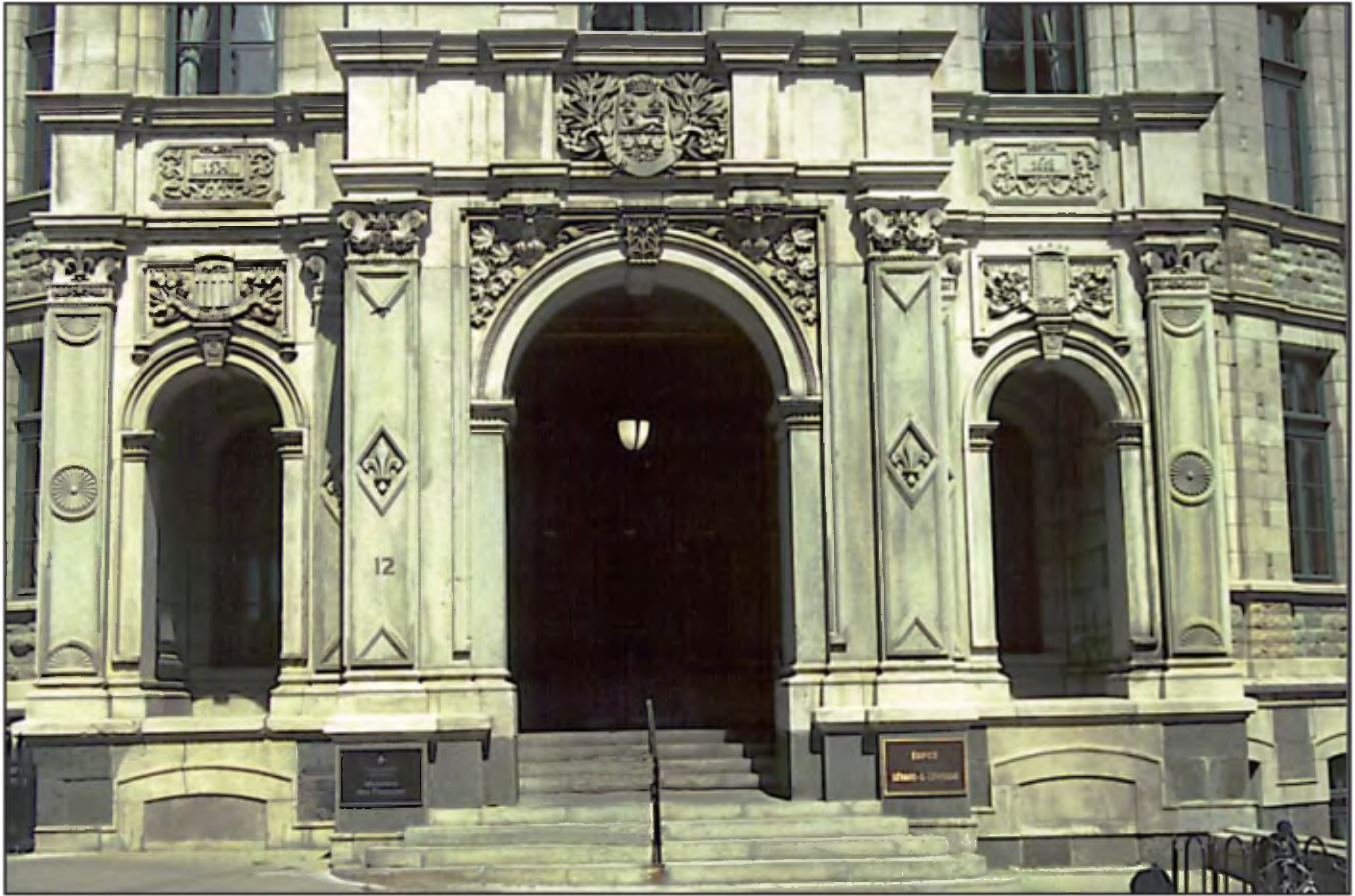
Portico of the former Court House of Québec City: pilasters in Stanstead grey granite; arcades, tympanum, coats of arms and capitals in Deschambault Formation limestone from Saint-Marc-des-Carières; footing in “Caledonia” granite from Rivière-à-Pierre replacing green Sillery sandstone.
