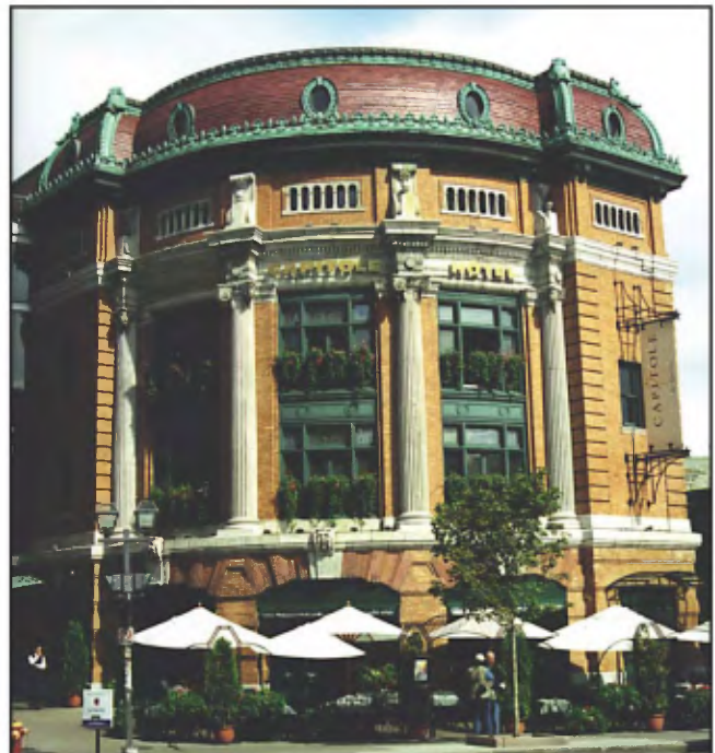
Théâtre Le Capitole: façade in bricks with Saint-Marc-des-Carières limestone trimmings and original slate roof.
