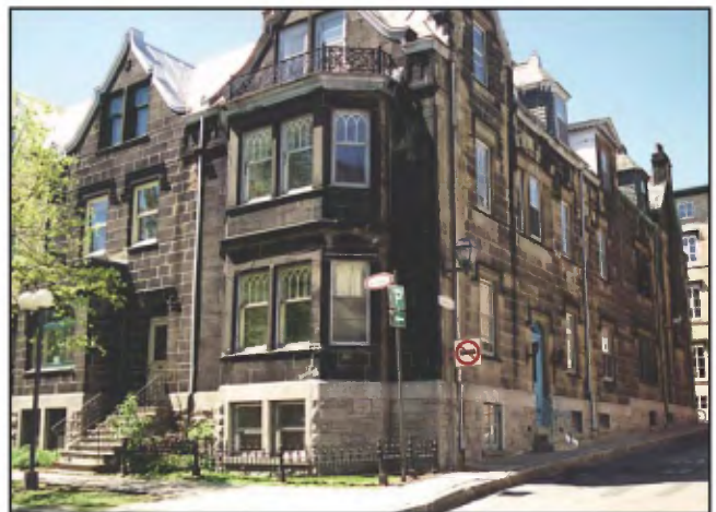
16, rue de la Porte, built in sandstone from Bouctouche area in New-Brunswick, with base in Deschambault Formation limestone.
