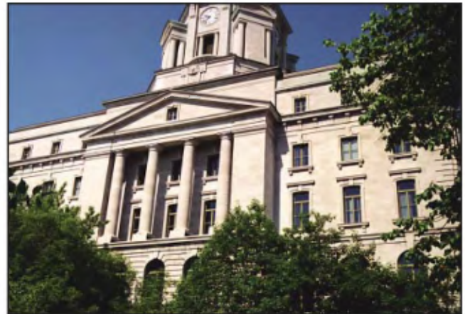
Louis-S.-St. Laurent building: facade and dome facing the river, built in 1913 with Deschambault formation limestone, quarried in Saint-Marc-des-Carières.
