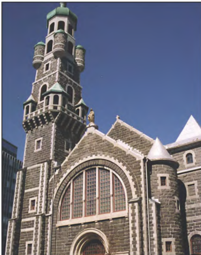
Saint-Coeur-de-Marie Church built in grey-pink granite from Rivière-à-Pierre and Deschambault limestone from Saint-Marc-des-Carrières.
