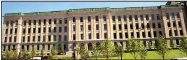
Honoré-Mercier Building: base in red gneissic granite, ground floor in grey-blue granite from Rivière-à-Pierre and upper floor in Deschambault limestone from Saint-Marc-des-Carières.
