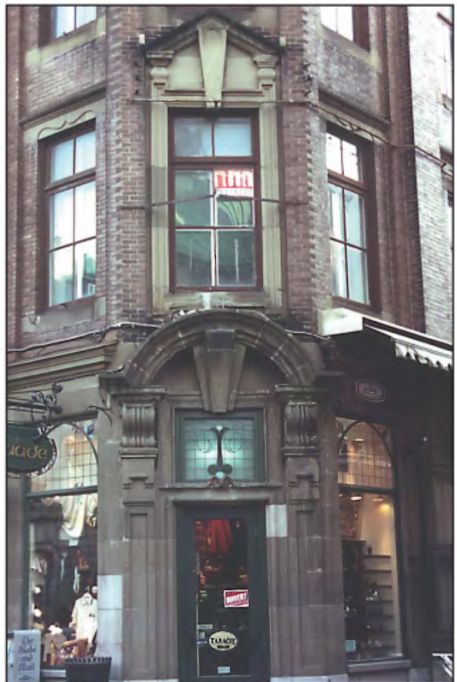
Corner facade of Daily Telegraph Building dresses with olive-green Miramichi sandstone.
