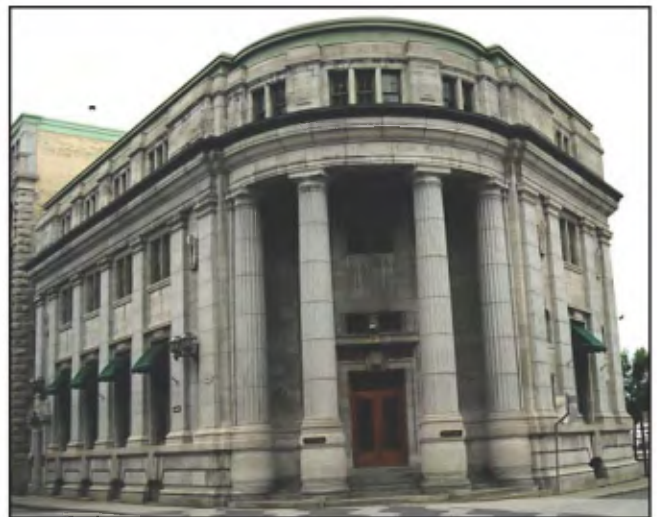
Former Bank of Commerce at 139, Saint-Pierre, with columns and pilasters in Stanstead granite, the rest in Deschambault limestone from Saint-Marc-des-Carrières.
