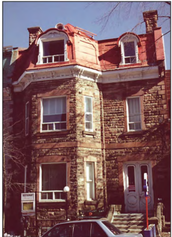
Building in white, pink and red sandstone from the Robitaille Formation, Lac Saint-Mathieu.
