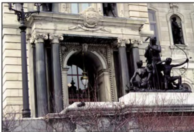
Portal of the honor entrance of the Parlement Building with columns in Quincy granite, capitals, vault, tympanum, cable moulding and walls in Terrebonne limestone, entablature in Deschambault limestone, and on the right the Halte en forêt Monument.
