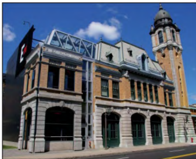
Ex Machina Theater: first floor facade on Dalhousie street in Saint-Marc-des-Carières limestone and imitation limestone fibreglass.
