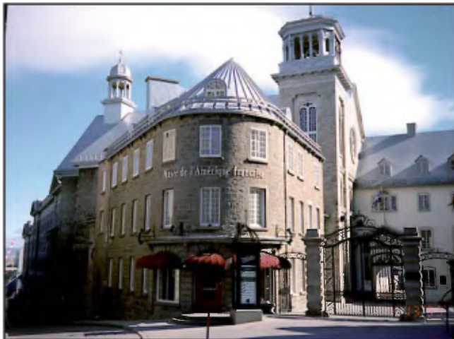
Musée de l'Amérique Française in Sillery sandstone from the Nappe de la Chaudière. The columns supporting the wrought iron gate are made of Deschambault Formation limestone from Saint-Marc-des-Carrières (see p.3).
