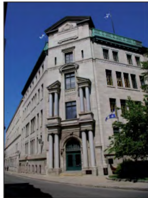
Corner front of 20 Pierre-Olivier-Chauveau street in Deschambault limestone and columns in Stanstead granite.
