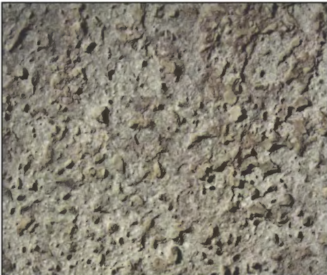
Honeycomb alteration in dolomitic limestone of the Chazy Group, Château-Frontenac.
