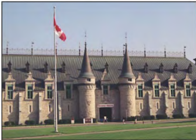
Manège Militaire on Grande Allée, built in Beauport limestone, Trenton Group, with limestone ornaments from the Deschambault Formation in Saint-Marc-des-Carrières.
