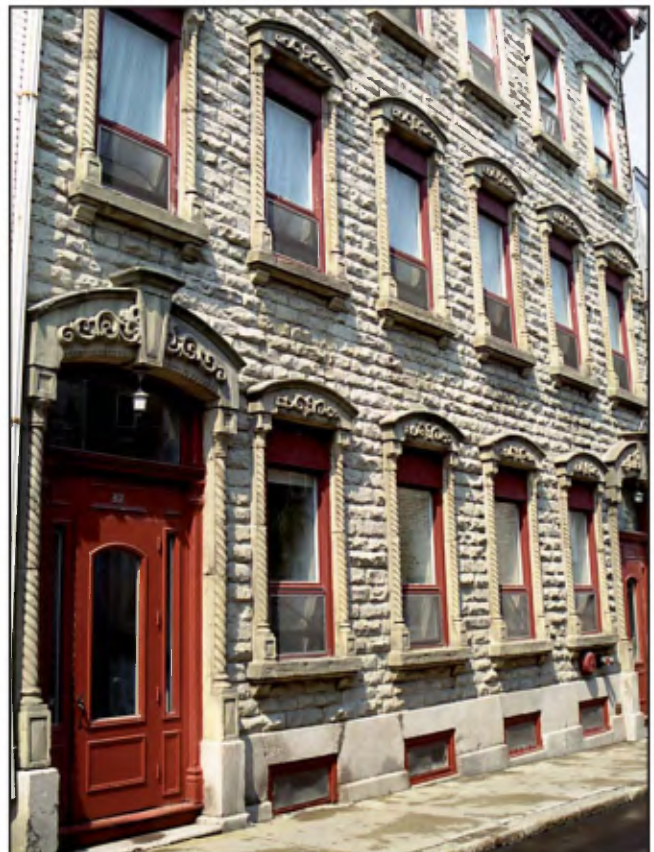
Maison Owen Murphy: front wall in La Malbaie sandstone, window and doorway frames in Ohio sandstone. Base in Deschambault limestone.
