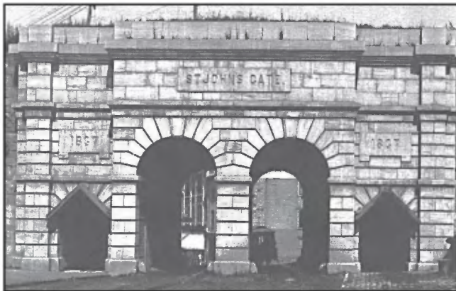
St. John's Gate built in 1867 with cut stones of Deschambault Formation limestone, when tramways were pulled by horses (Notman archives).
