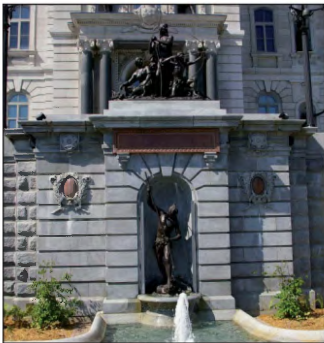
Niche of “Pêcheur à la Nigog” sculpture in moulded limestone blocks from the Deschambault Formation in Saint-Marc-des-Carières, overlain by a lintel of red granite from St. George, New Brunswick.
