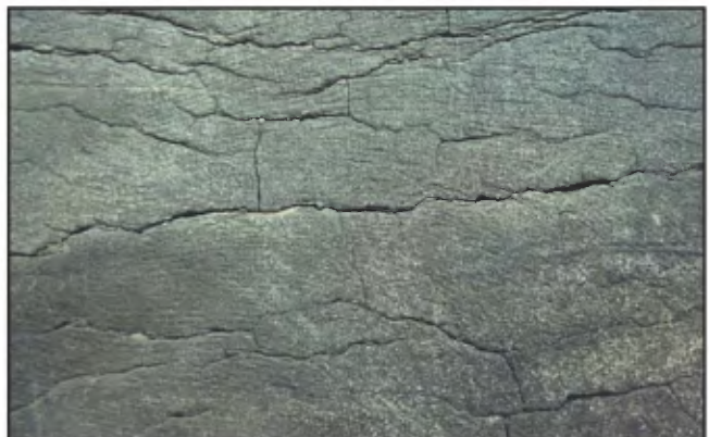
Fracturing along stylolites in Pointe-aux-Trembles limestone on the Wolfe-Montcalm Monument.
