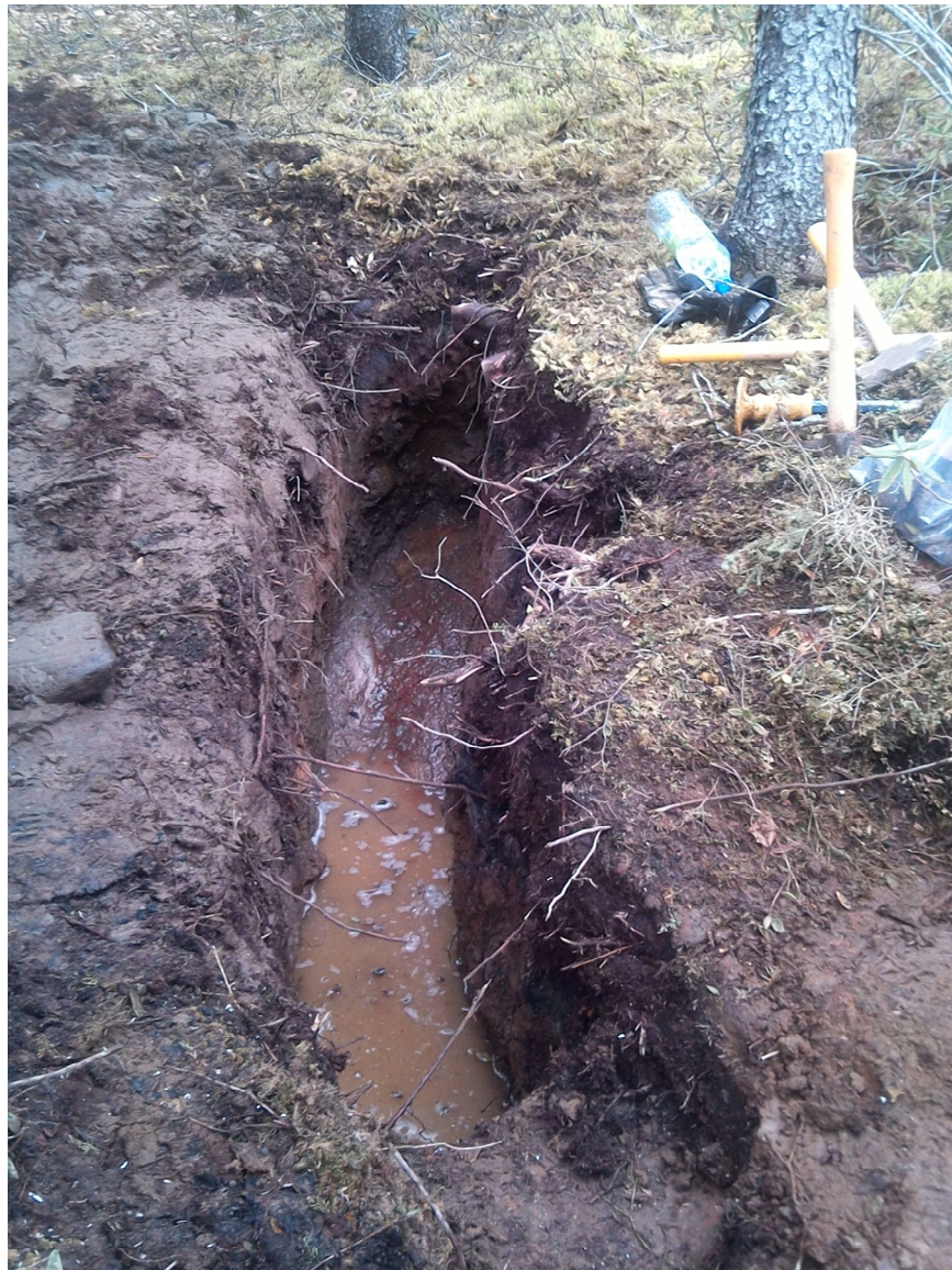
Photo 4: Shovel-dug trench at the GEM Zone.
