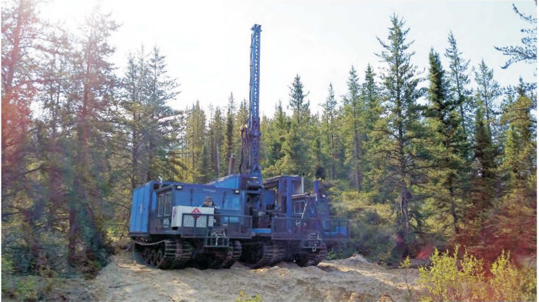
Figure 15 - RC drill rig and support vehicle at Hole 18.
