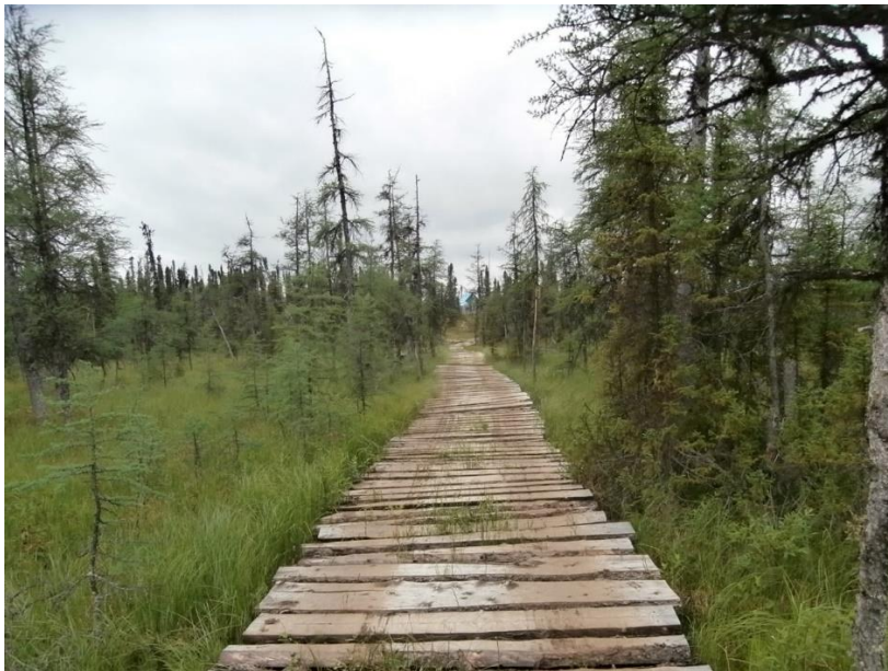
Figure 7-12 Crossing, made of wooden planks, over swampy area at start of main trail
