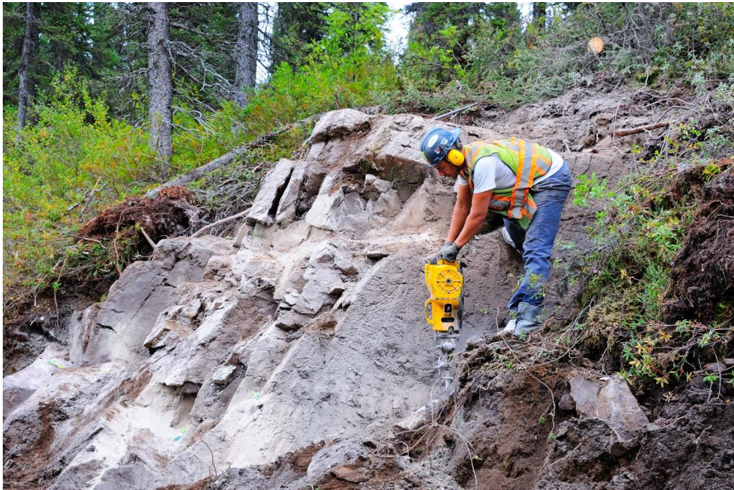
Figure 7-7 Bulk Sample Site Pre-blasting
