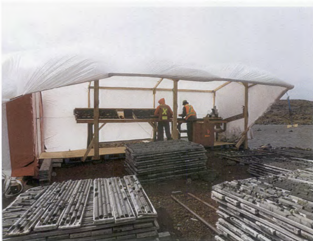
Picture 2: Temporary core shack at Twin Lake, Kyak bloc.
