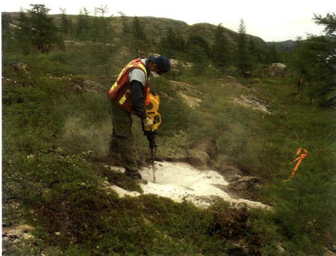
Picture 9: Site preparation for "Boulder buster" with a Pionjar rock hammer.
