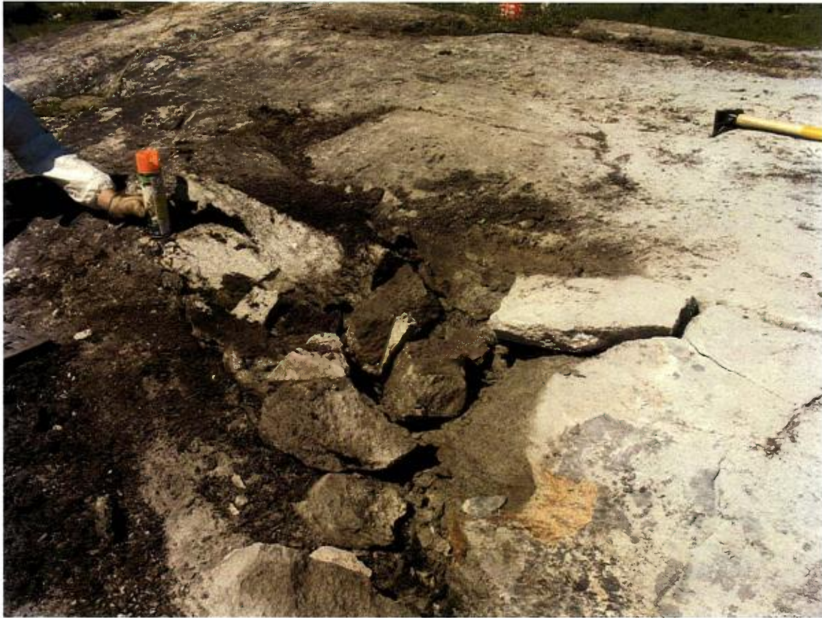
Picture 10: View of a blasting site using "Boulder buster".
